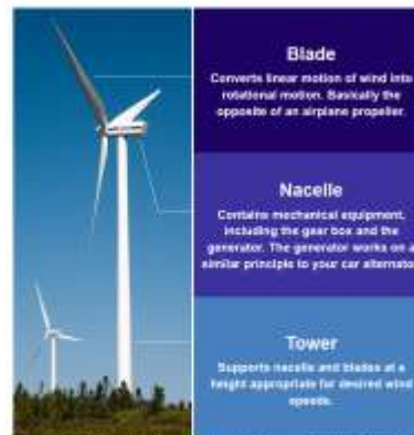
Pictou Point wind turbines located in Yarmouth County — 1.6 MW, 263 ft (118 m) Image released under the Creative Commons Attribution-NonCommercial 2.0 license by the author.
